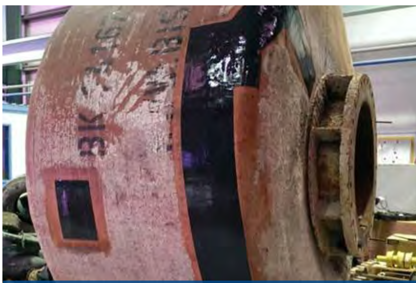
Damaged areas repaired
