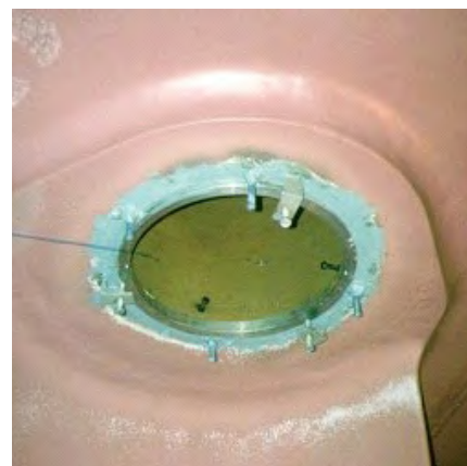
Rudder bearing bonding - bottom view
