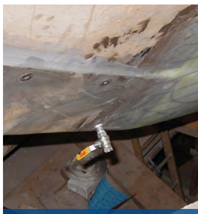
Anchor pocket bonding in progress
