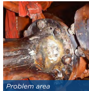
Live leak sealing
